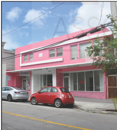
1950 Moderne Office, 1034 NW 3rd Avenue
