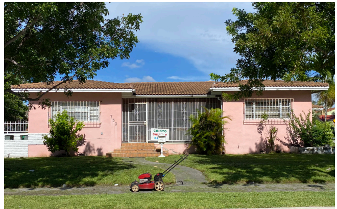
This one-story Ranch-style home, built c.1950, features a low-slope hip roof with spanish tile and overhanging eaves, an incised open entry porch, a built-in-garage, slump brick details and built-in planters.
