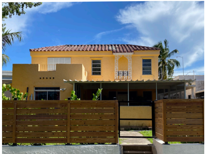
Photo 19. 1511 NW 9 Street, construction of an aluminum screened porch in the front yard. (Image Source: Plusurbia Design)
