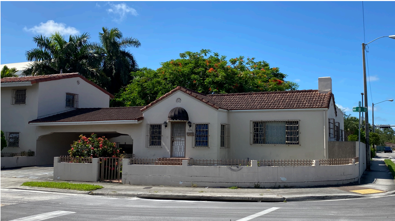
Photo 04. 1646 NW 8 Street. (Image Source: Plusurbia Design)
