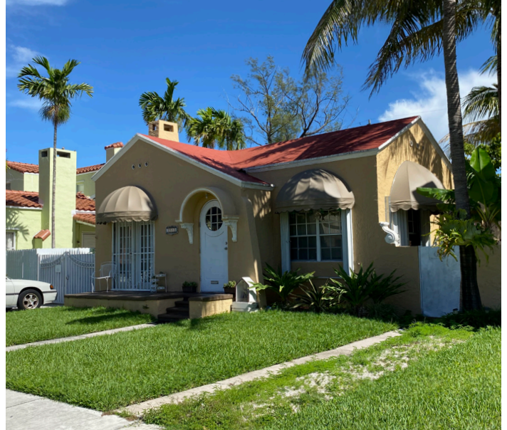
Photo 15. 1533 NW 8 Street. (Image Source: Plusurbia Design)
