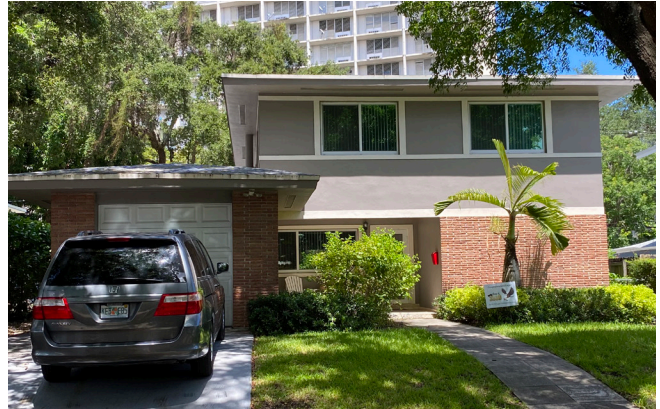
This two-story home, built c.1950, is an unusual example of Prairie style in Miami and in its mid-century time period. It is notable for its horizontal lines, the applied brick at the ground level, and continuous sill line below the 2nd-story windows.
