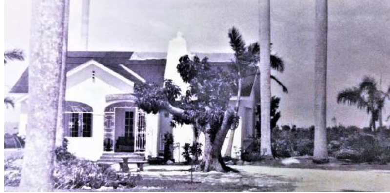
The Forbes/Juan Gabriel Historic Site after Hurricane Andrew, 1993
